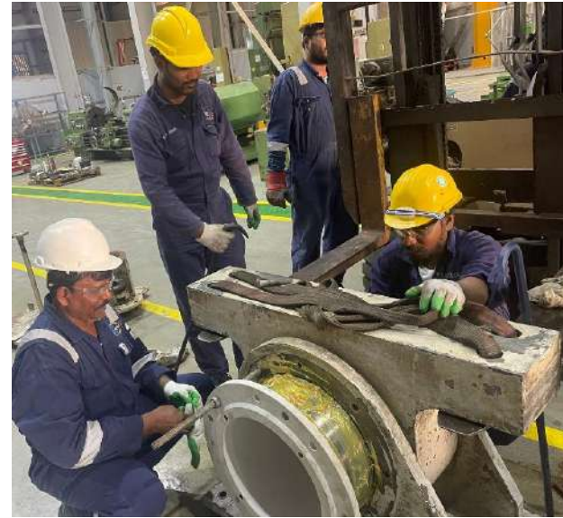
Components Maintenance /Replacement at site
